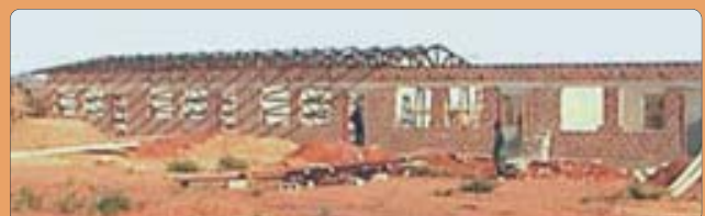
Framing the roof
