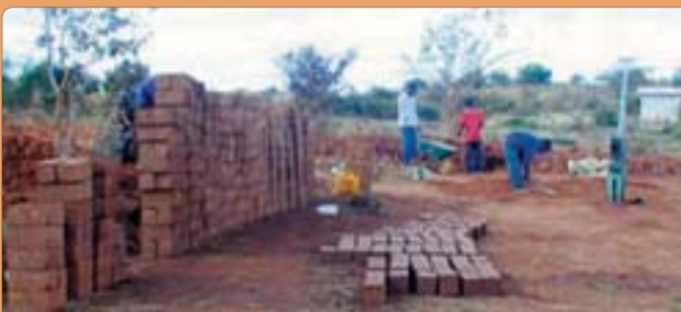
Ready to build
