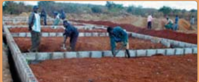
Foundation almost complete
