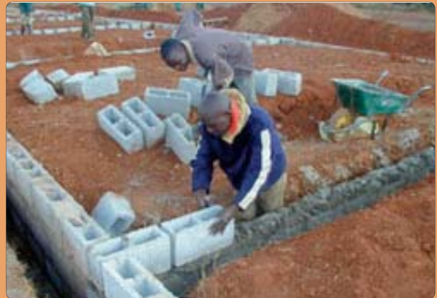
Setting the foundation
