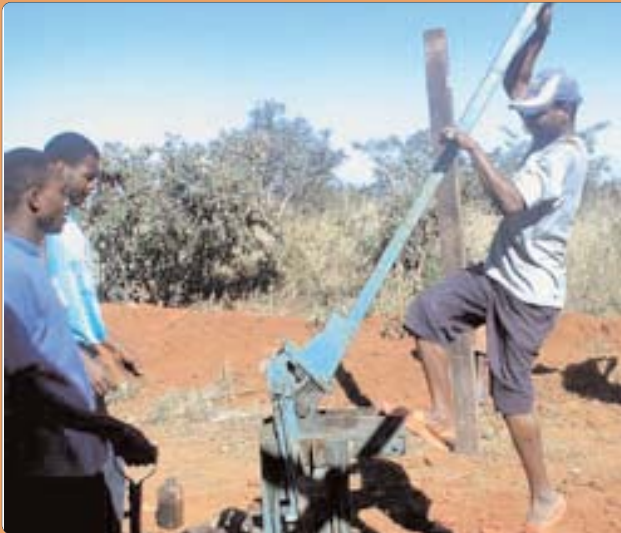
Getting the block press going
