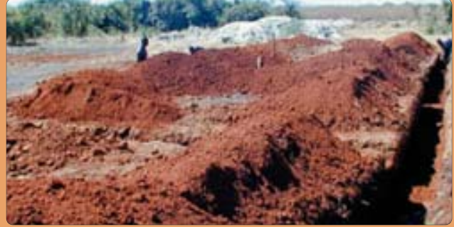
Ready to begin laying the foundation
